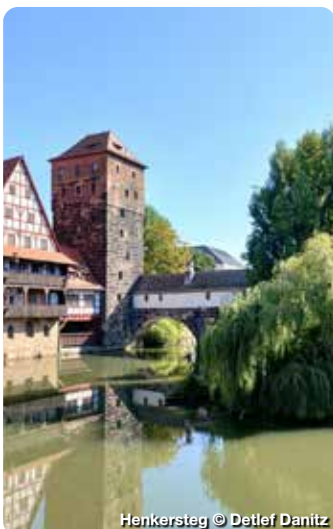
Henkersteg © Detlef Danitz
