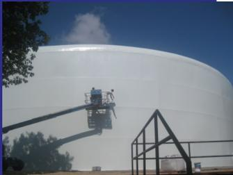
Coatings applied to the water storage tanks provide a protective barrier between the steel and the moisture in the atmosphere.
