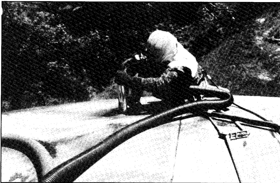
Vacuum blasting of lead-based paints on the exterior of a water storage tank will control atmospheric emissions. (See related story, page 7.)
