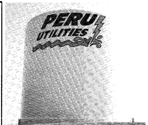
New 1,000,000 gallon tank Peru Utilities
