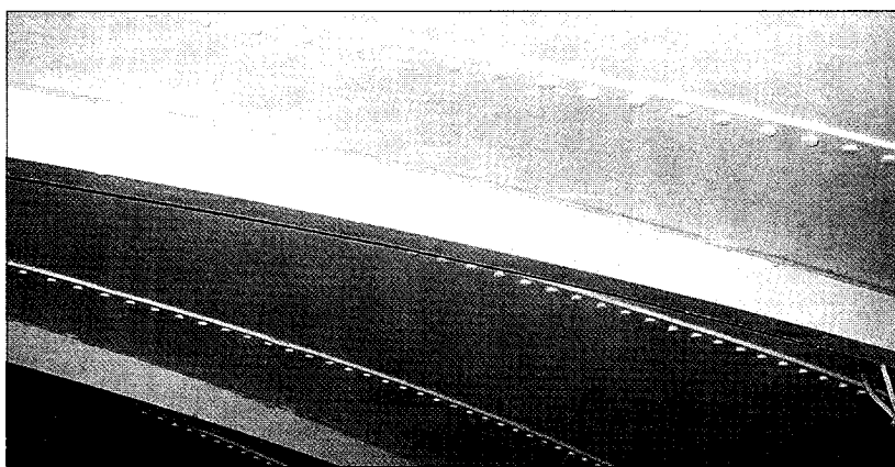
■ (top) Blast cleaning the outside of the bottom of a riveted elevated tank
