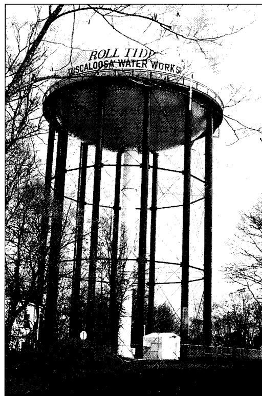
■ Courtesy of Tank Industry Consultants and Tuscaloosa Water Works
