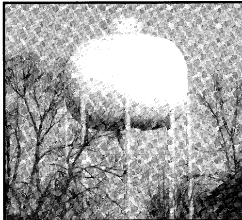
Antenna installations can be concealed as on the roof of this multi-column tank. Photo courtesy of Stealth Network Technologies.
